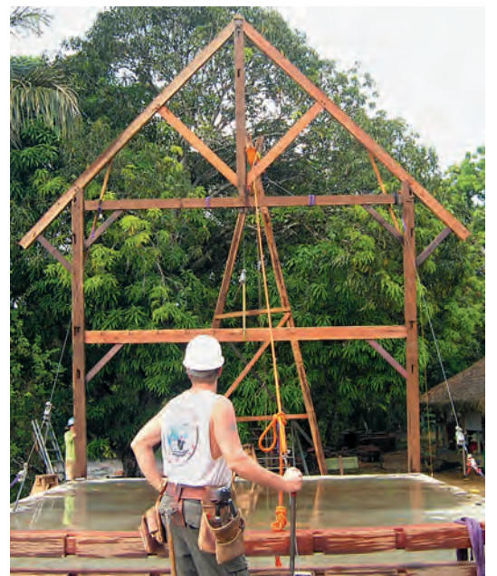
Steve Lawrence Fig. 9. Bent 12 raised with help of A-frame.
