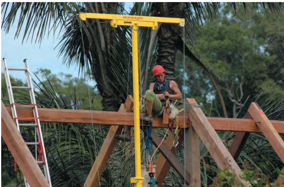
Fig. 8. The indefatigable, indispensable, fully rigged Adrienne Walker, setting rafters.
