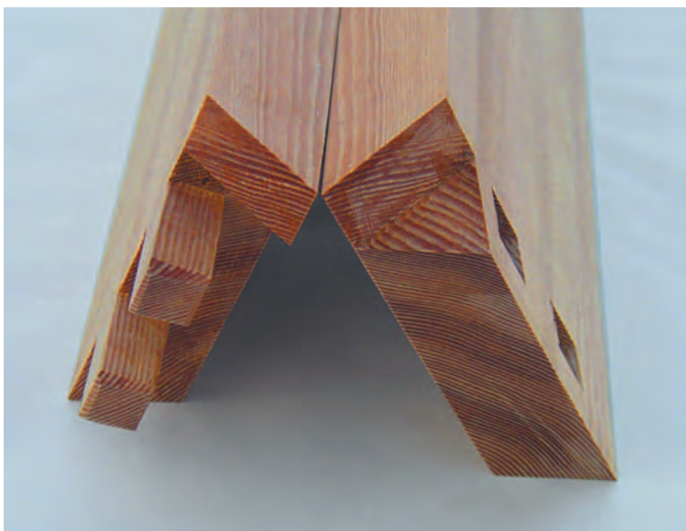
Fig. 5. Mortises, tenons and miters cut at ends of hopper boards.
