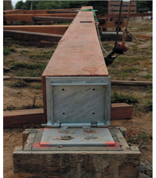
Photos Anne Phillips except two below Fig. 7. Close-up of hinged hold-down for post.
